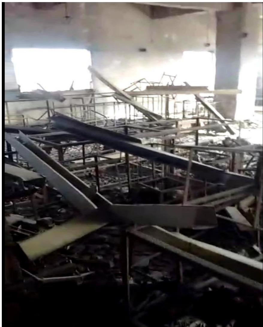
The illegally built mezzanine floor of the ill-fated Ali Enterprises
